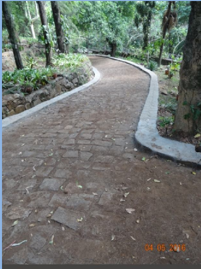
Renovation of pathways
