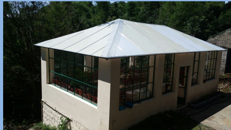
Green House renovation
